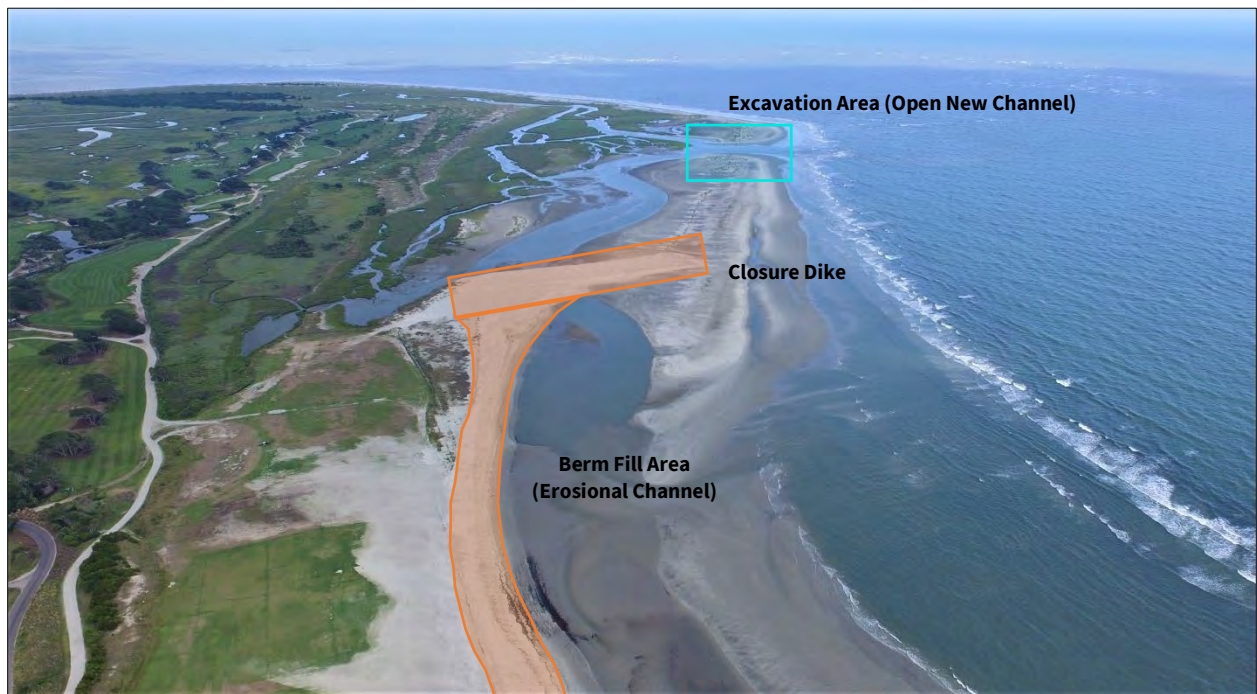
FIGURE 2.10. [UPPER] Excavation and fill areas used in the 2015 project. Approximately 100,000 cy of sand was transferred from the excavation area to the fill. [LOWER] Project area on 7 July 2015, after project completion, showing closure dike in the center of the image and a new flushing channel at the upper right. Encroachment by the ‘erosional channel’ destroyed hundreds of feet of dunes, leaving no protection in front of the driving range.
